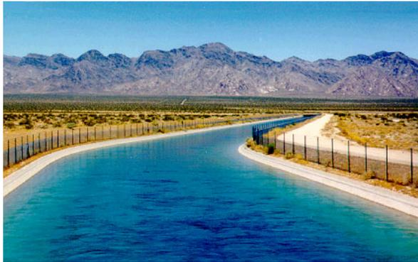
Figure No. 4. The Colorado River Aqueduct Hinds Pumping Plant is at the base of the mountain in the background
