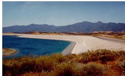
Figure No. 2. Lake Mathews Main Dam Concrete lined upstream; rock on downstream face (almost 1.2 km. long)
