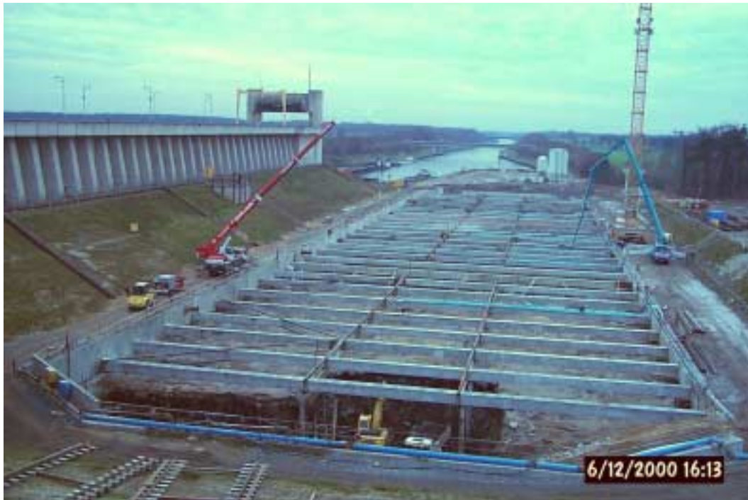
Figure 2: Panoramic view of the building site
