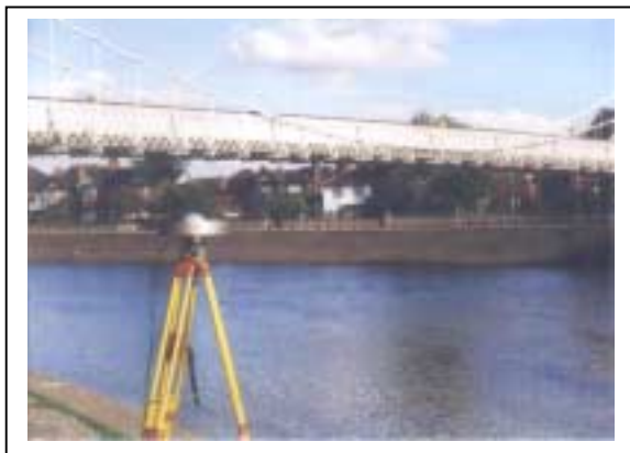
Figure 6 Nottingham suspension footbridge over River Trent.
