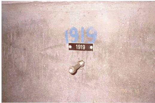
Figure No. 4 Control point in Tunnel Insert with adapter mounted.
