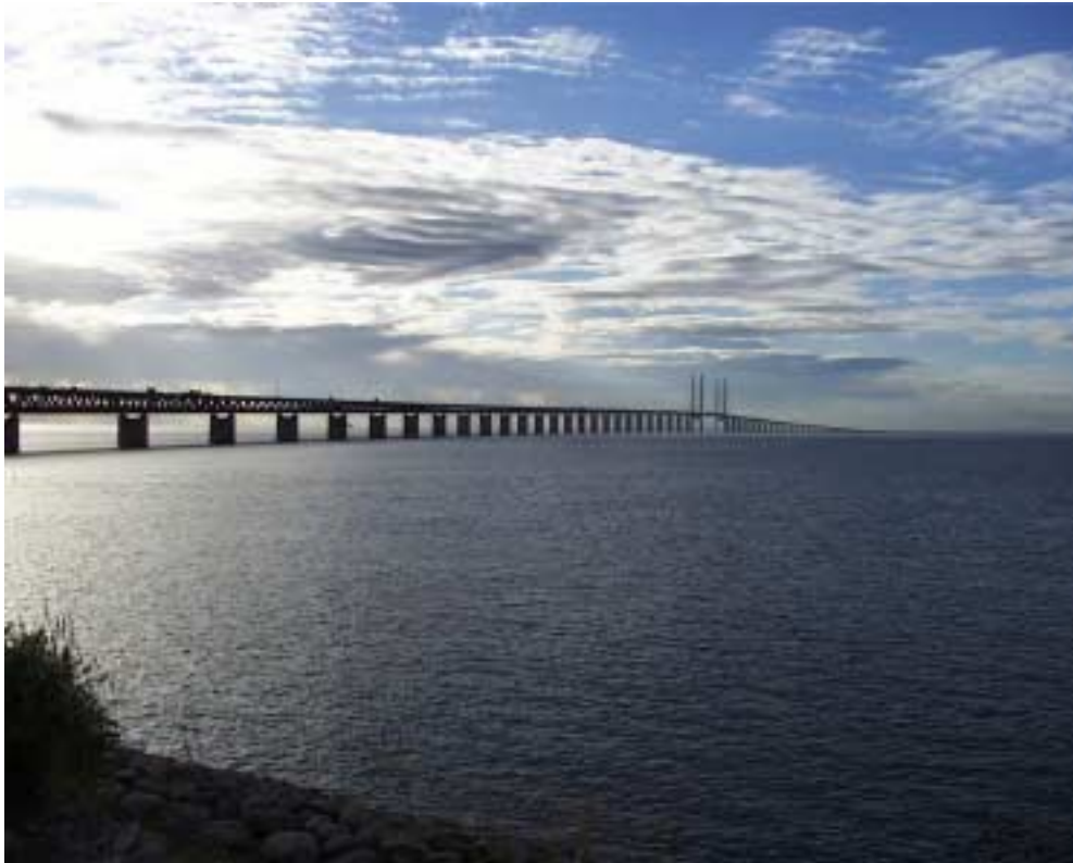
Figure No 2. The bridge seen from Sweden
