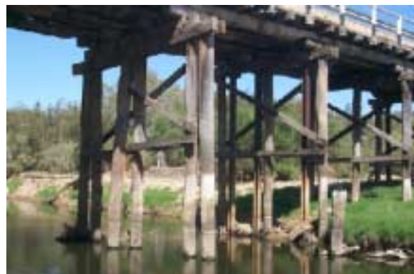
Figure 5: Photograph of a section of Toodyay Bridge.
