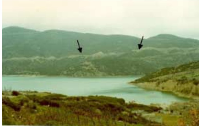
Figure 2: The ‘Beta’ landslide, view from south. The road is shown in fig. 4.
