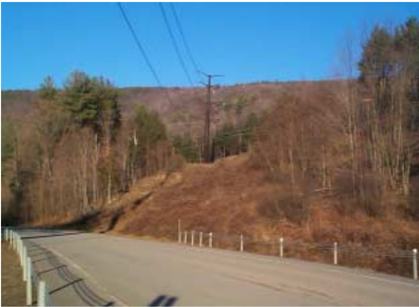
Photo 1. Northeast view of the slide in upstate New York. Note the hummocky terrain associated with landslide topography. Station REM1 is just beneath the tower.
