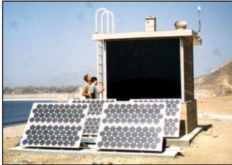
Figure 6. Observing station TS4, on the West Dam
