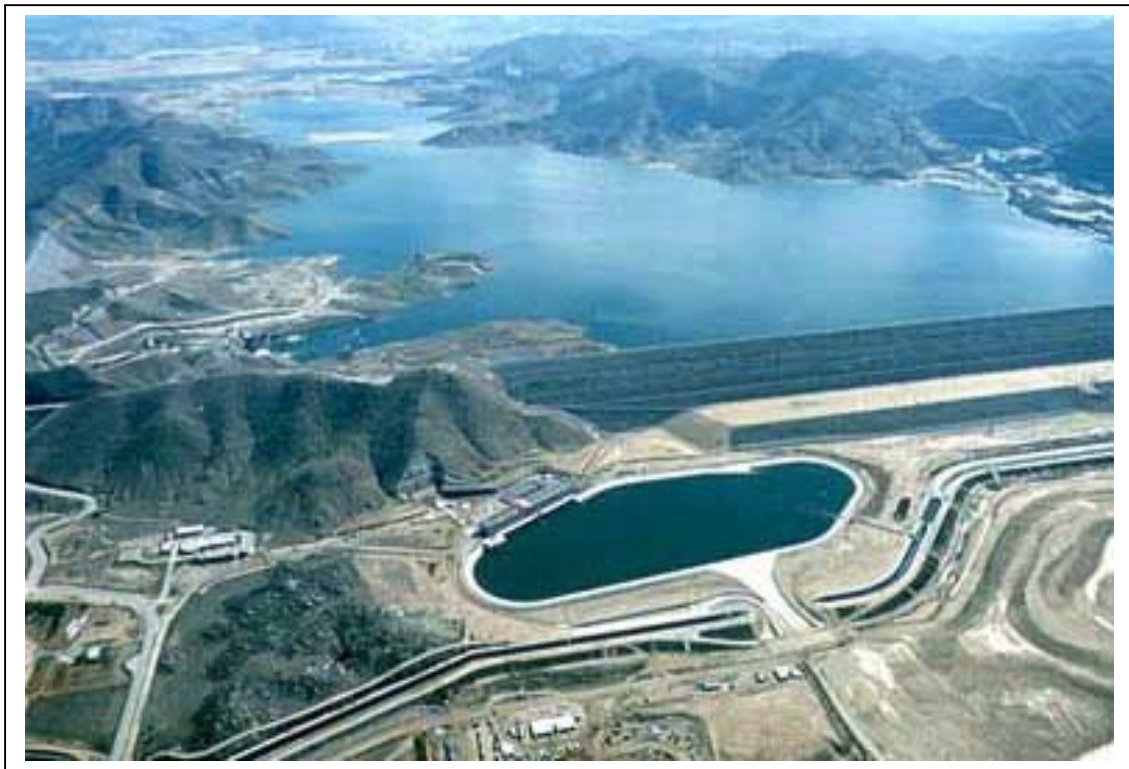
Figure 1. An aerial view from the west of Diamond Valley Lake in Riverside County. With a surface area of 4,500 acres and a storage capacity of 800,000 acre feet (260 billion gallons), the reservoir will provide six months of emergency supplies in the event of a major earthquake, provide additional water for drought protection and peak summer needs, and nearly double the region's surface water storage capacity ( Metropolitan Water District of Southern California , http://www.mwd.dst.ca.us/ ). Shown is the northern end of the West Dam and the smaller Saddle Dam. The West Dam is monitored in real-time by two Leica CRS1000 receivers, the Saddle Dam by one receiver. Altogether seven Leica CRS1000 receivers and AT303 antennas are deployed on three large earthen dams and at two reference sites located on stable rock close to the two larger (West and East) dams. (See Figure 2 for a map view of the GPS network).
