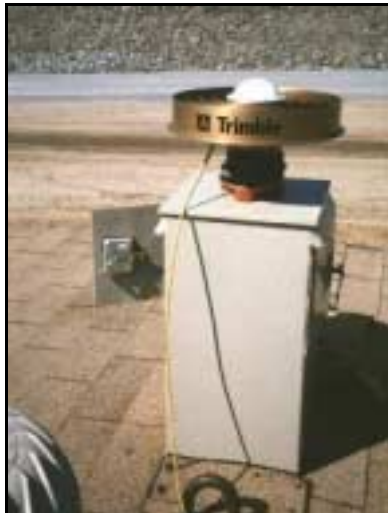
Figure 7. Choke ring antenna on observation shelter roof.
