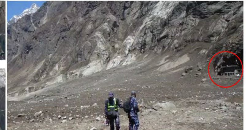
(b) Just one house was left standing in Langtang after the landslide
