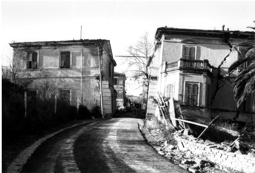
*Fig. 1 direct impact caused by a landslide*
