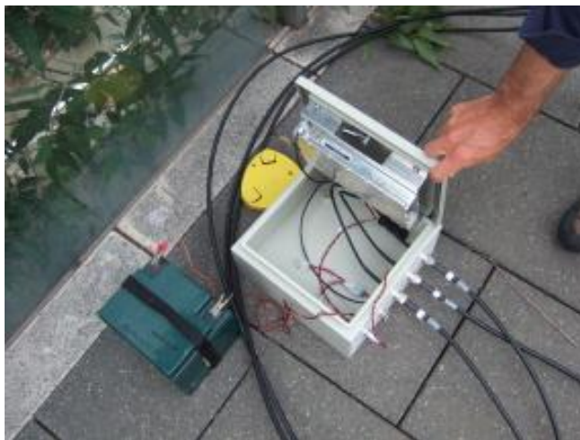
Figure. 1a: LocataLite inside box with cabling to antennas.
