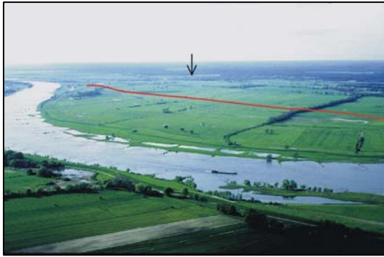
Fig.9: the run of the new dyke
