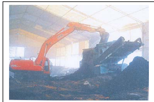
Treating of contaminants (soils) within a building. www.groundscience.com Source: Environment & Earth Science International
