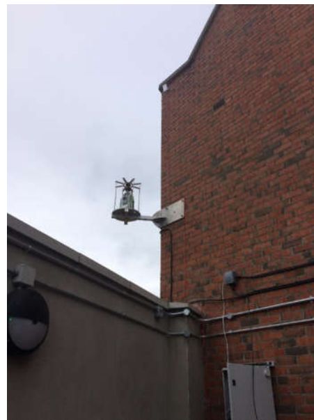
Figure 5. Difficult set up installation.
