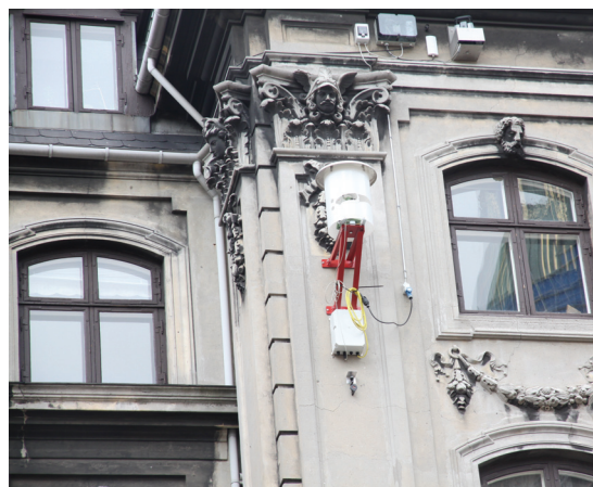
Fig. 3 Automated total station on building facade.
