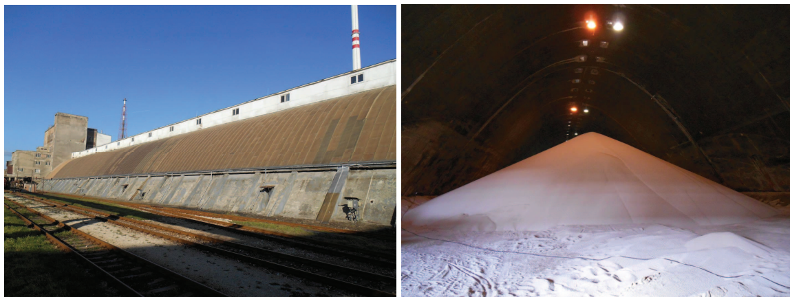
Figure 1 The construction of the warehouse
