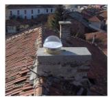
**Fig. 7**: Type 1 – Pedestal on the concrete base
